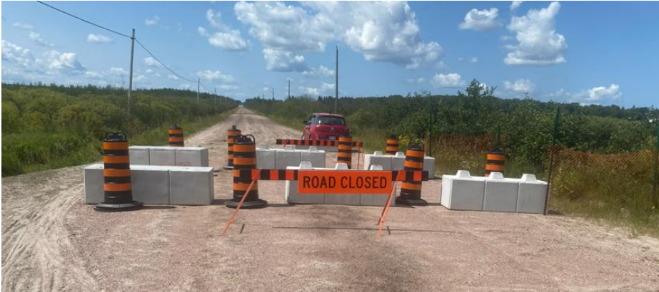
Current road closure setup by Township Public Works staff at Culvert Failure
