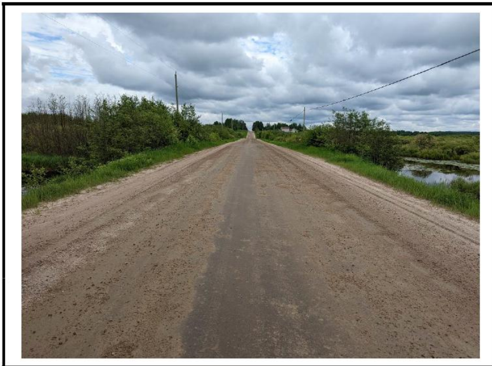
Photo 2 Structure from west approach
