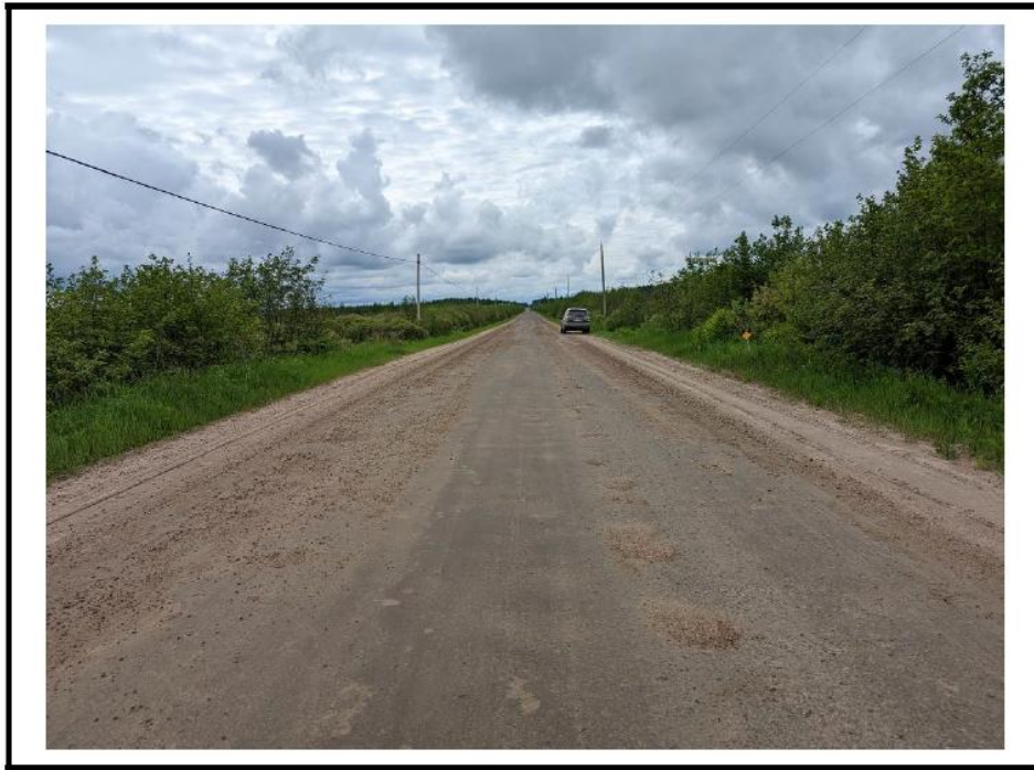
Photo 1 Structure from east approach
