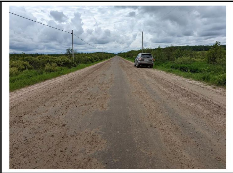
Photo 4 West approach from centre of structure
