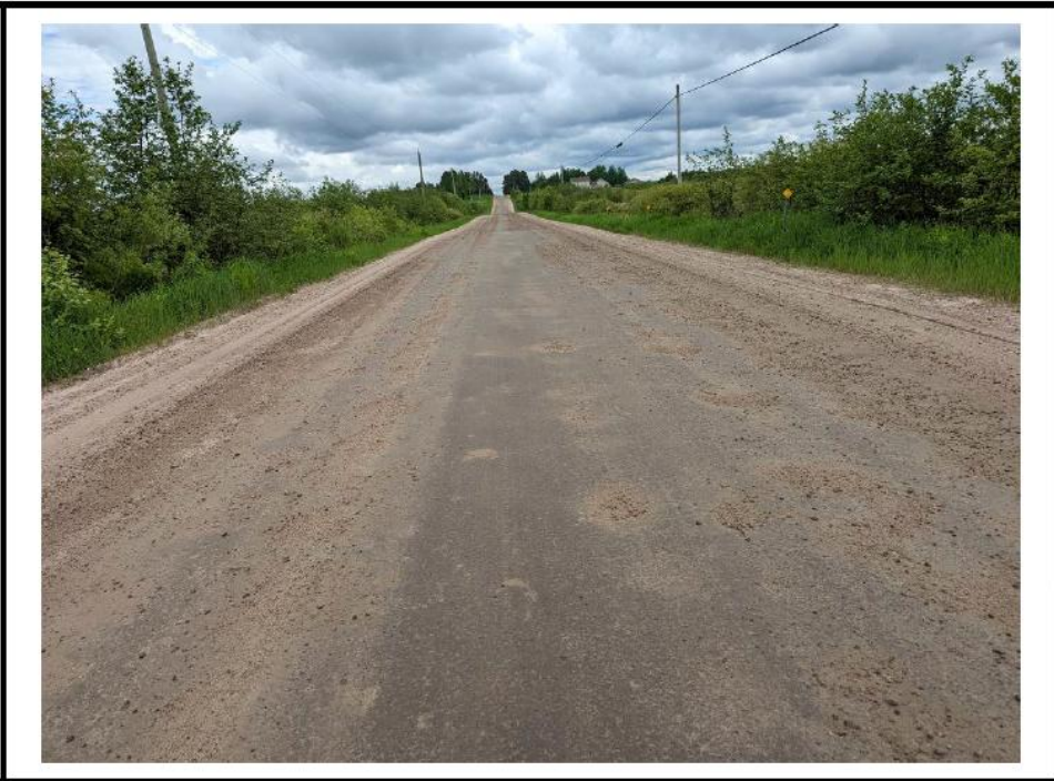
Photo 3 East approach from centre of structure
